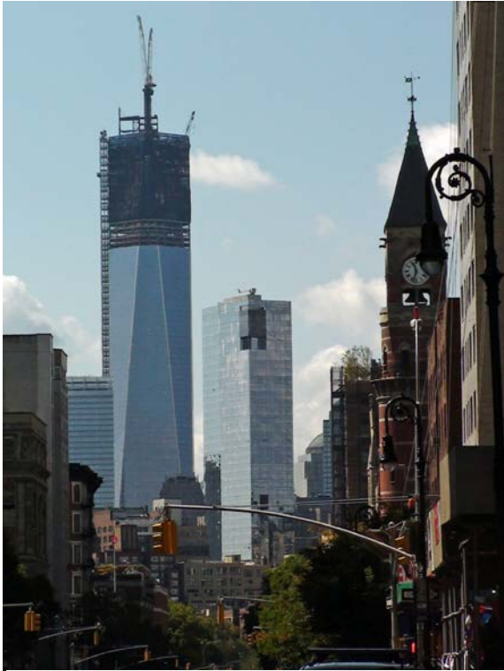
The new World Trade Center Tower 1 under construction 10-4-09
